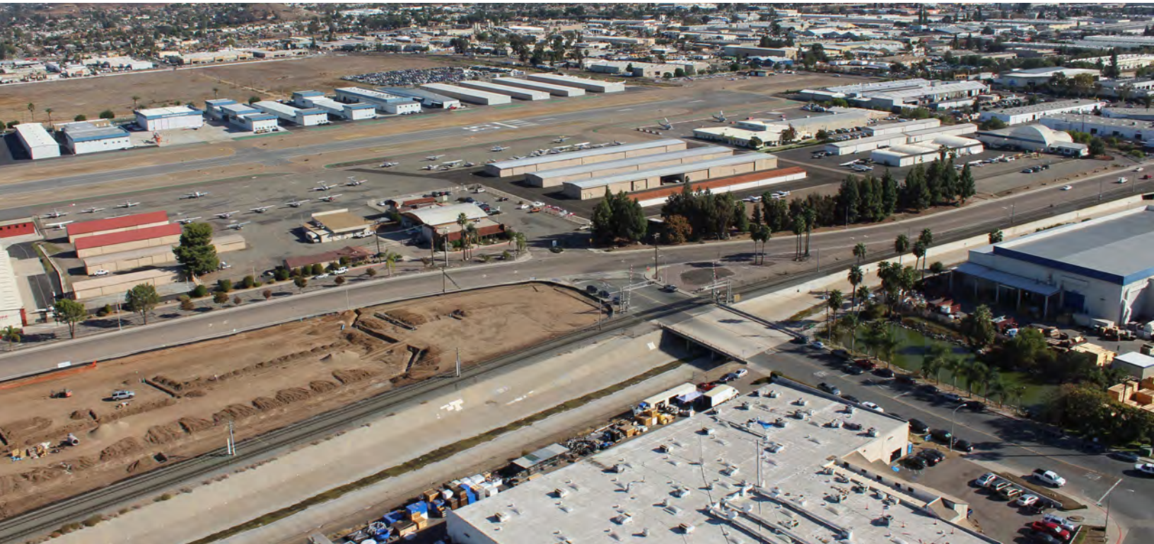
Figure 4.28 Aerial of Forester Creek System: industrial area in El Cajon, Forester Creek in foreground with view to Gillespie Field
