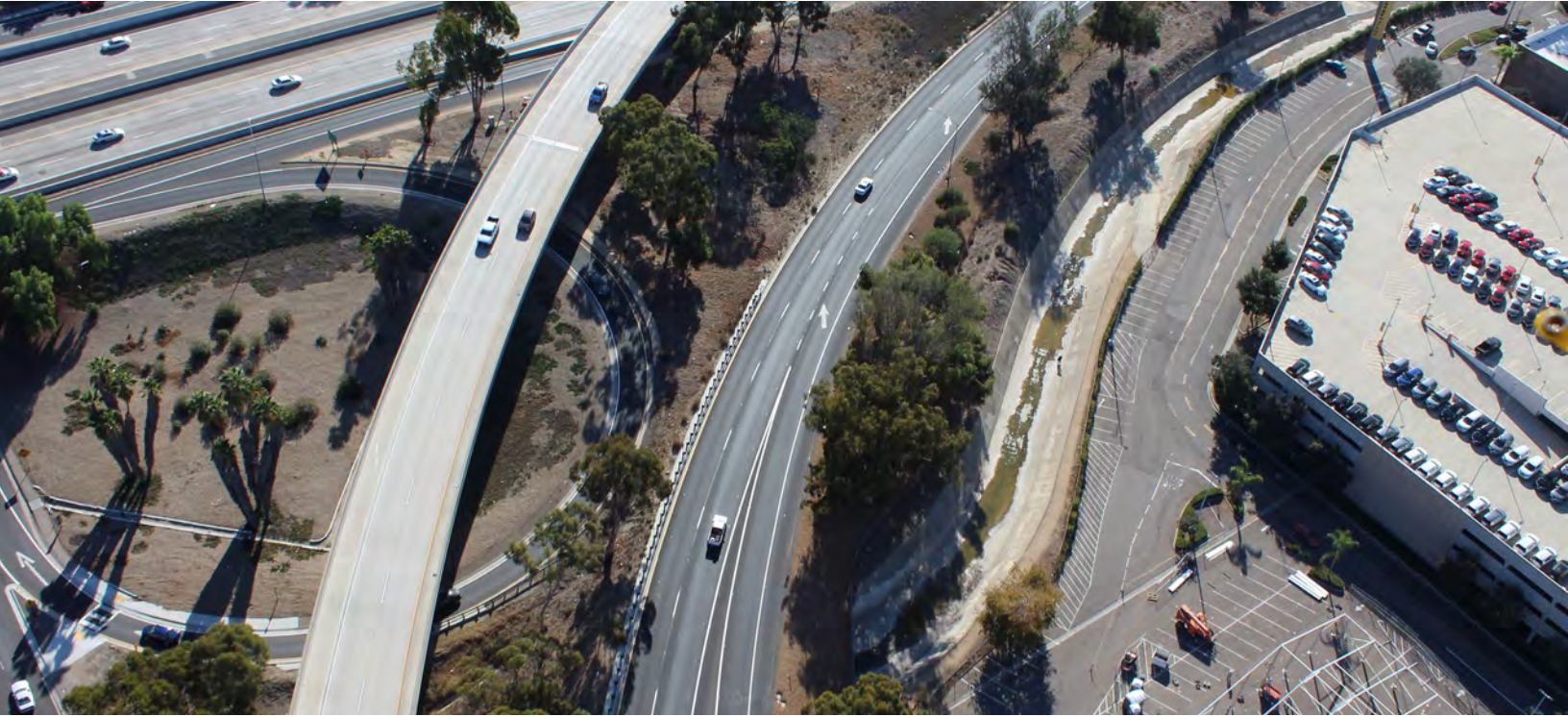
Figure 4.27 Aerial of Forester Creek System: Highway 67 and 8 interchange at Parkway Plaza
