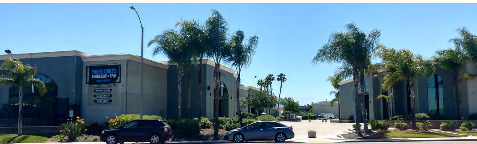
Figure 4.01 Land uses adjacent to Broadway Channel
