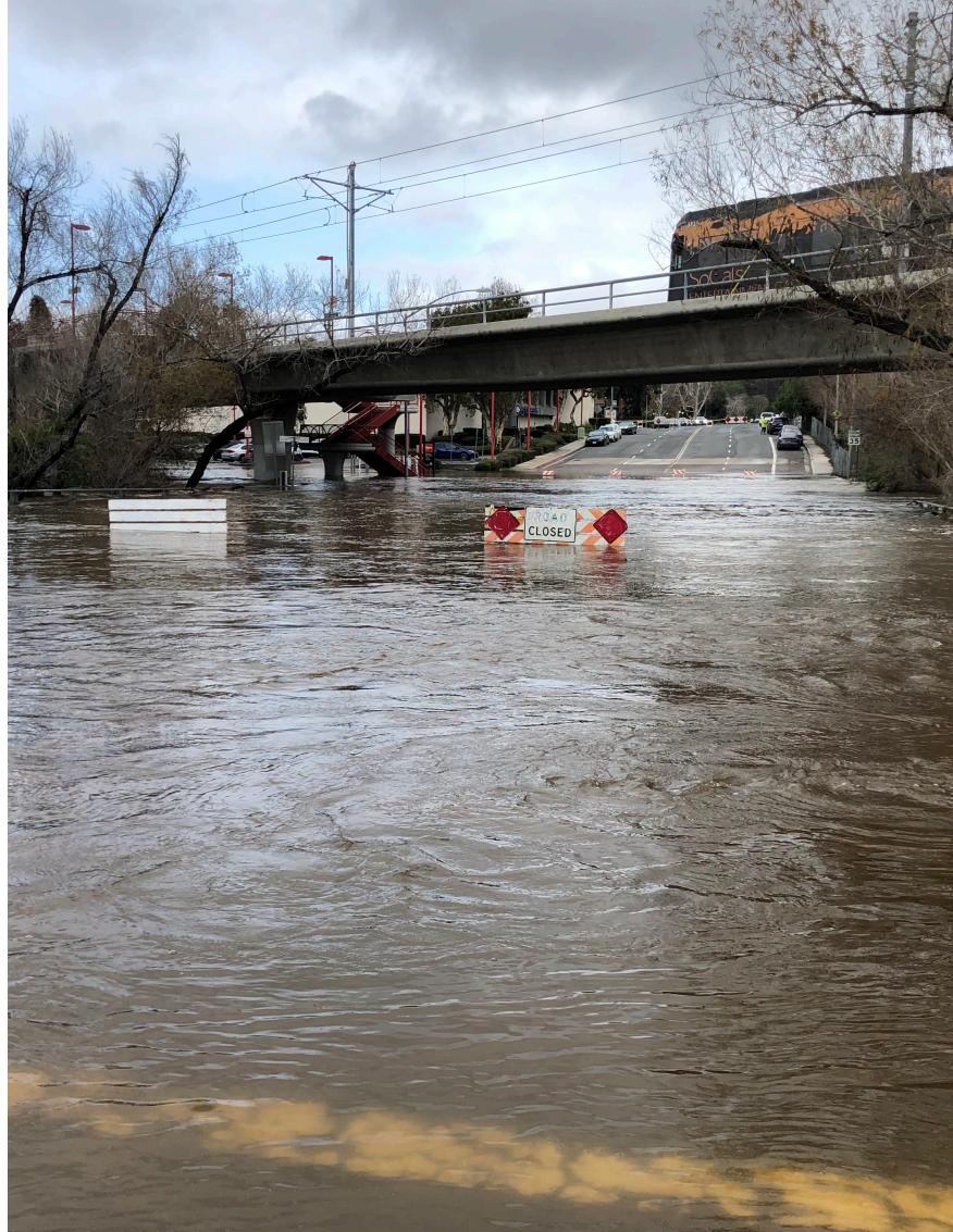
Stormflows at Fashion Valley Rd., downstream of WQM Site 3
